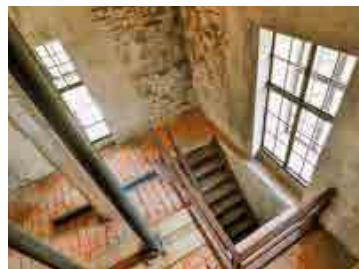
Interior of the Water Tower
